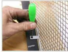
Install Step #14: Now mark upper & lower mounting tabs. (this process will insure a proper fit)
