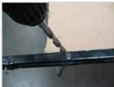
Install Step #34: Drill 3/8 hole into metal support bracket.
