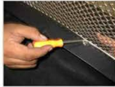
Install Step #29: Mark grille mounting tab center hole locations using a sharp scribe.
