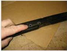
Install Step #16: A view of the holes drilled into grille shell support.
