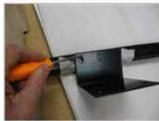
Install Step #14: Align latch bracket with tape lines as a guide and scribe latch bracket holes onto grille support.
